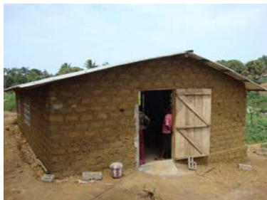
New Life Bible Church built within the last six months.
